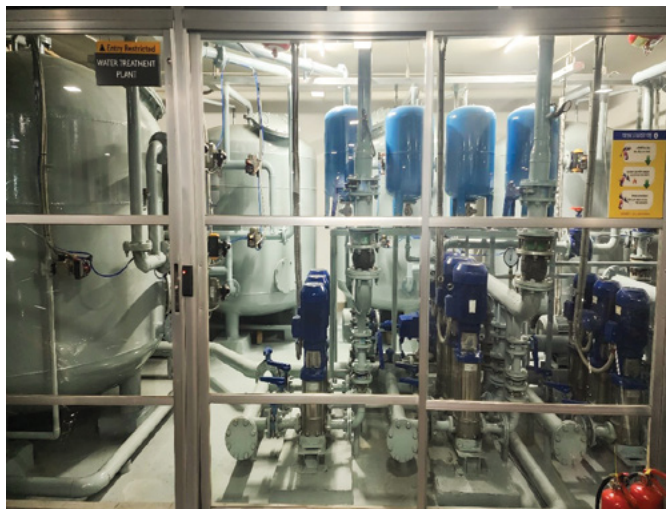
Water Treatment Plant
